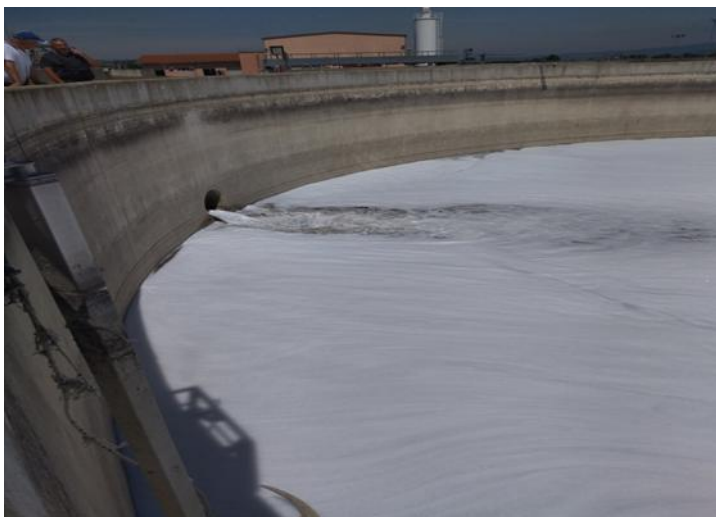
Slika 2. Ulaz deterdženta u postrojenje Figure 2. Detergent inflow into the plant
